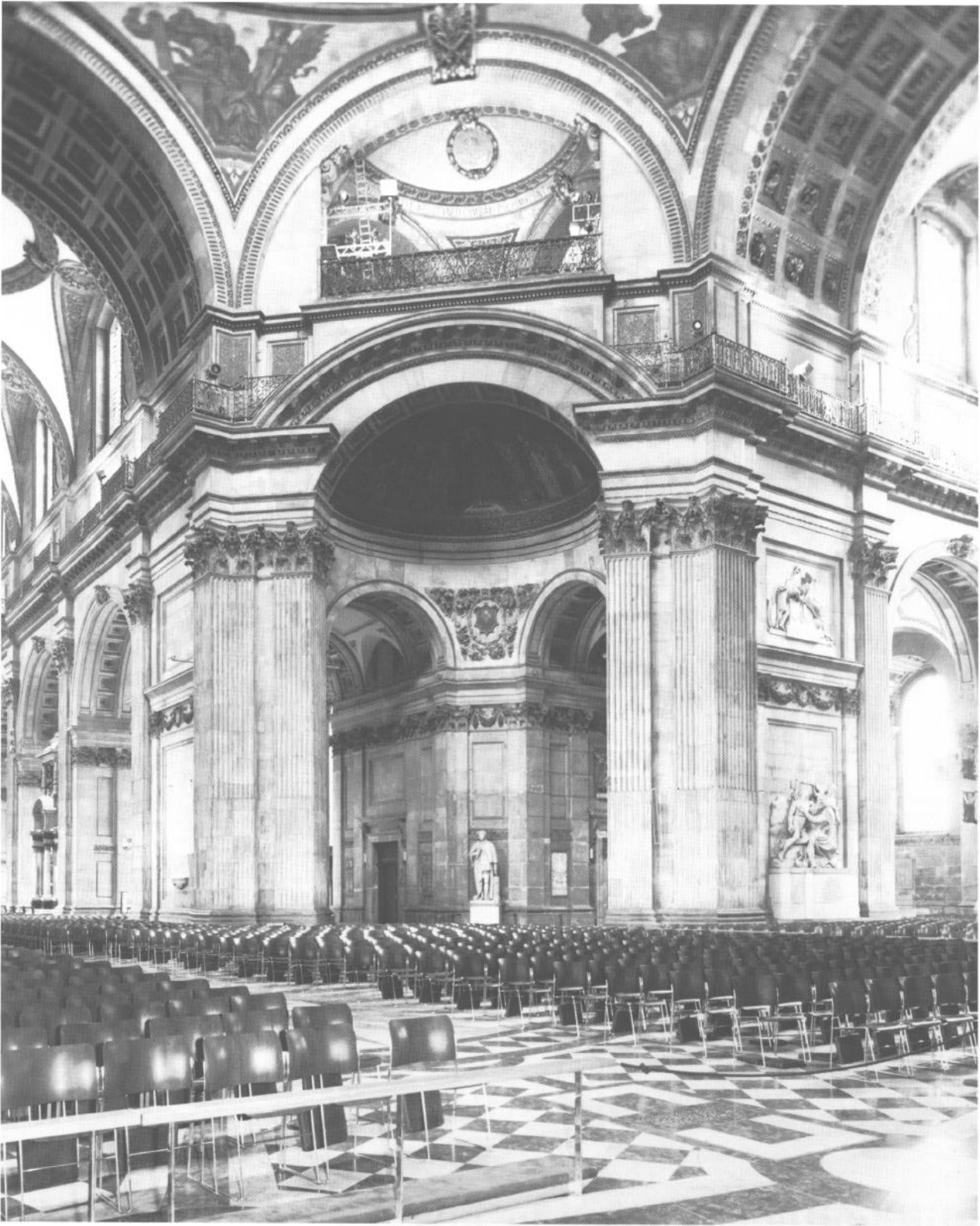
Fig. 12. Stone pillars which support the dome
